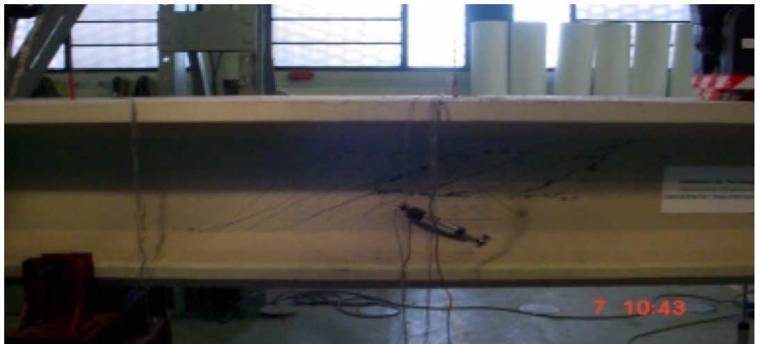
Figure 39: Case PB6. Details of the girder at failure. The picture is taken from (Choulli, 2005).
